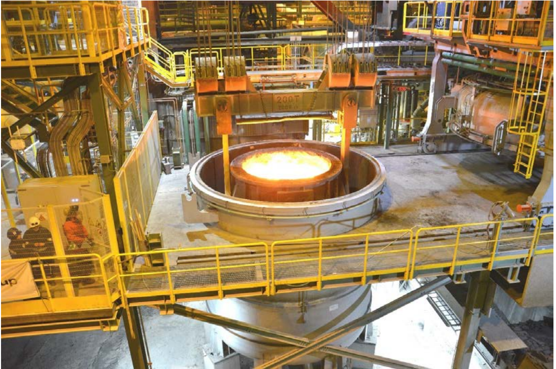
Station for vacuum treatment. The ladle is placed in a container, a lid is put on and air is sucked out while argon is bubbled through the melt. Negative pressure causes gases to escape from the molten steel.
