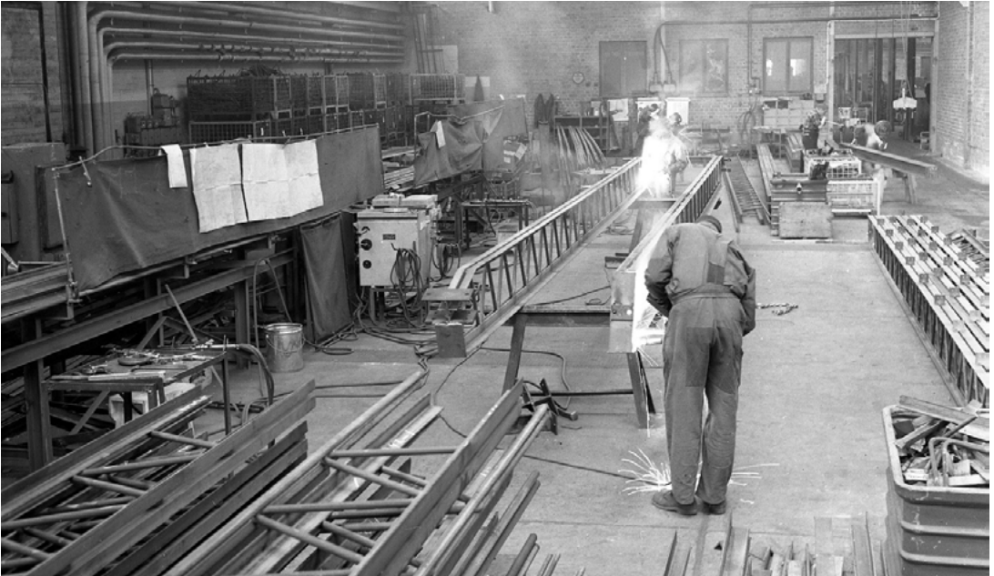
Welding of roof trusses.
