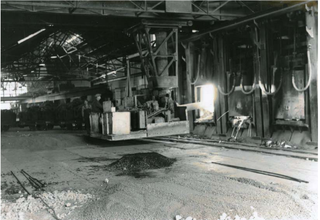
Insertion of scrap in Martin furnace No. 4
