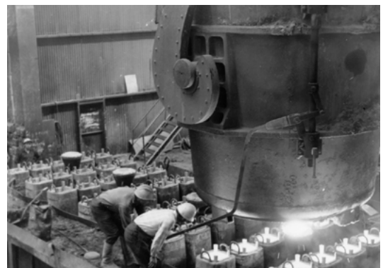
Casting of ingots by bottom pouring
