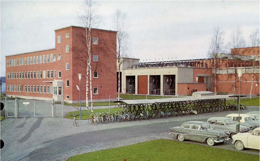
ASEA's High-Power Laboratory, inaugurated in 1958. Foto: Hitachi Energy
