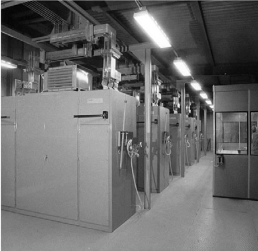
Thyristor compensator, SVC, in cabinets with cooling fans and heavy-duty busbars. Photo: Harry Frank
