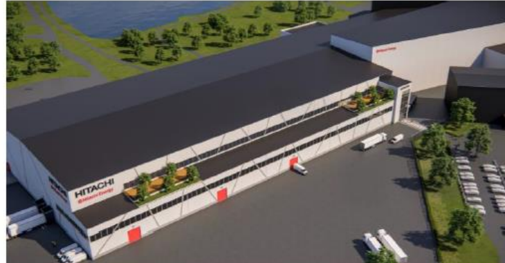
Transformers capacity, Ludvika
