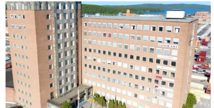
Renovation of main office, Ludvika
