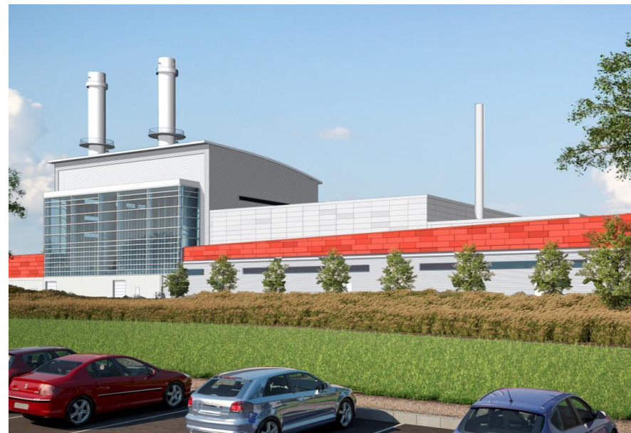
2 x SGT-800 Combined Cycle Plant supplying electricity and heat for City of Holland, U.S.A, replacing an old coal fired plant
